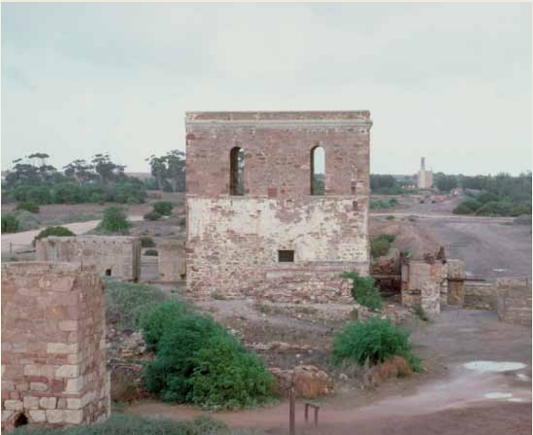
Cornish mining landscape, Moonta Mines State Heritage Area
